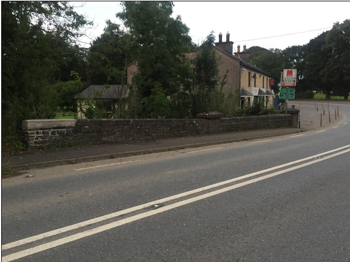
Plate 10.10: Crettyard Bridge (NIAH 12400605), looking north east
