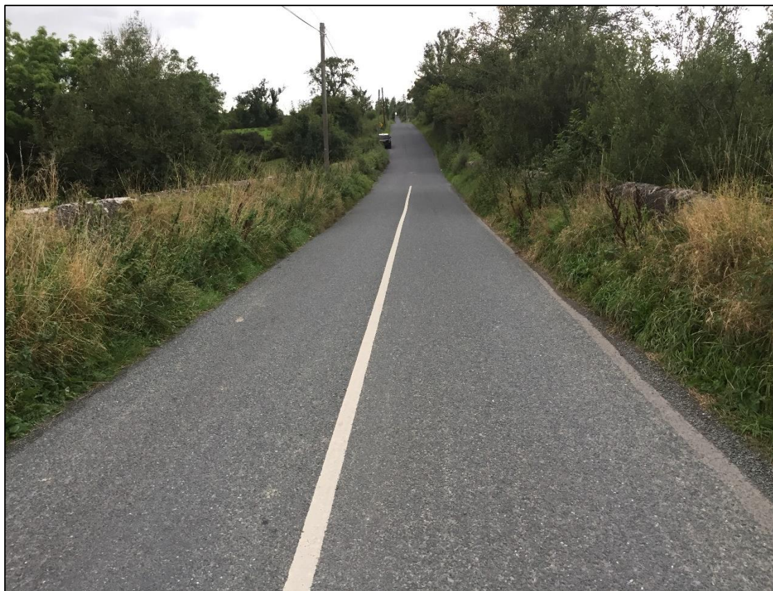
Plate 10.9: Black Bridge (RPS D84/NIAH 12401111), looking north west
